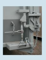
The ratchet latch tightens against the door seal and insures a tight seal.
